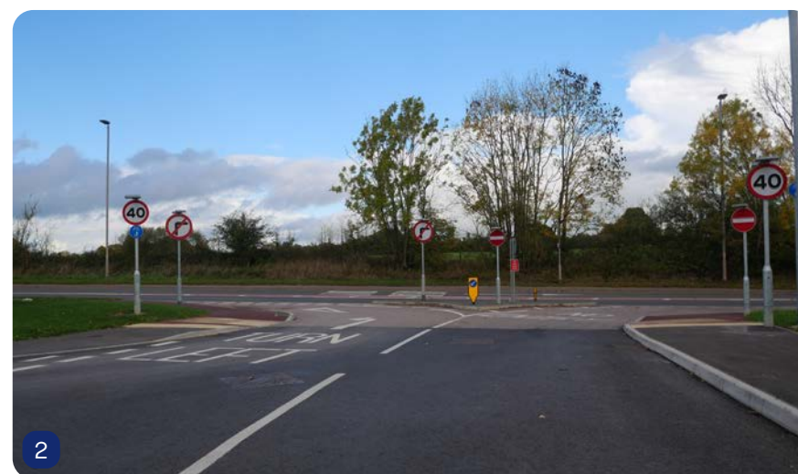
Taunton Road / Mount Vets junction and the site frontage
