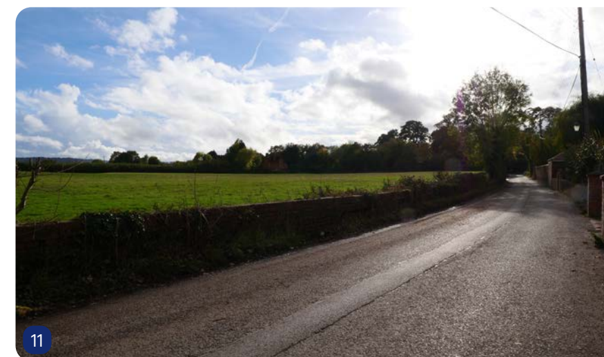
Poole Industrial Estate link road looking into the site
